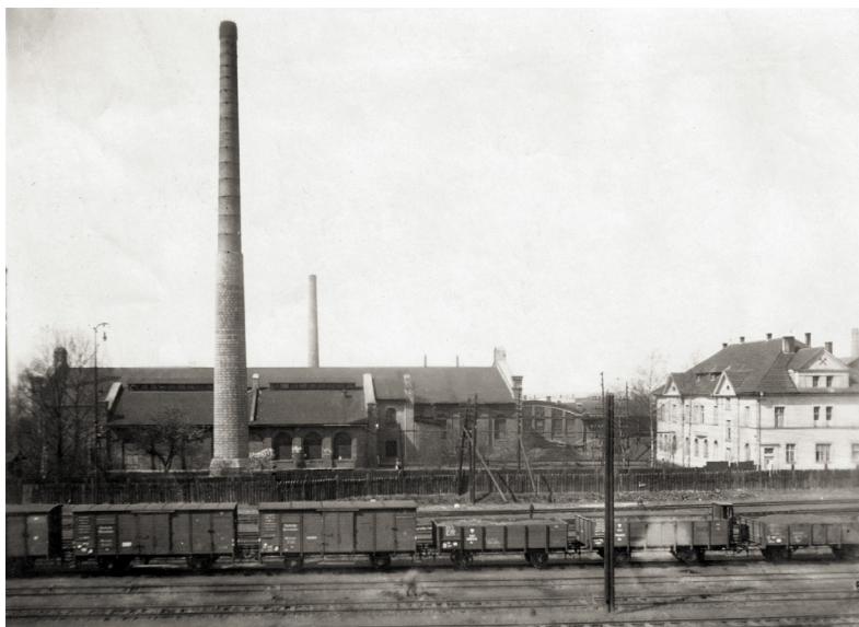
7. View of the metal rolling mill in Dziedzice from the south (ZAO, the unsorted fond of Válcovny kovů, a.s. Moravská Ostrava-Prívov 1851–1945 [Metal Welding Factory, Moravská Ostrava-Prívov])
